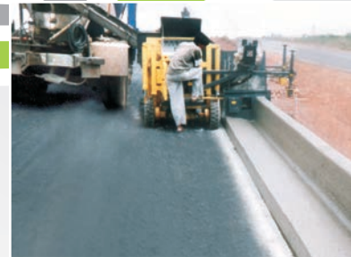
Super Elevation / Gutter Section
