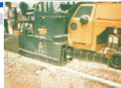
Kerb With Reinforcement
