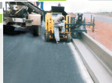
Super Elevation / Gutter Section
