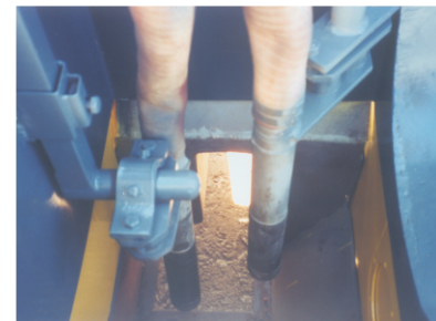
Needle Vibrator In Mould Box
