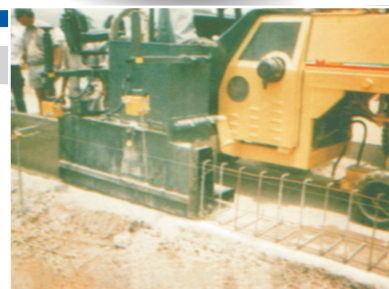
Kerb With Reinforcement
